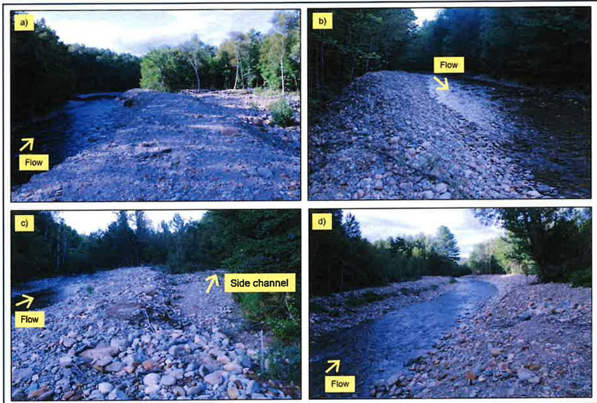
Figure 14. Four berm types constructed in December 2023: a) “in channel” berm (Rollins Site), b) “on floodplain” berm (Bennett Site), c) “blocking side channel” berm (Langdon Site), and d) “gravel veneer” berm (Langdon Site).
